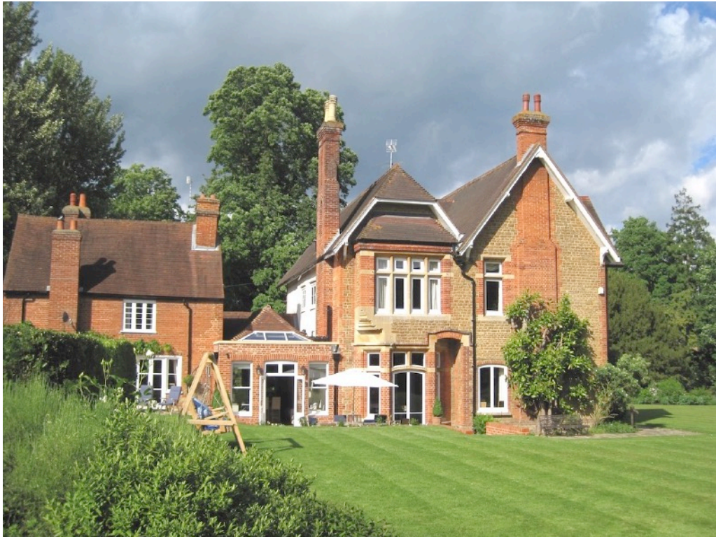
The south-east and south-west wings of the house were added by Rev William Davies in 1875.
